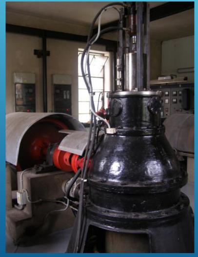
Kaplan turbine made by this company - the first installation of its kind in the world
